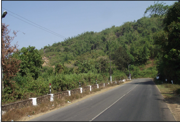
Photo 1: View of the NH-17 between Ankola-Karwar with Western Ghats at background
