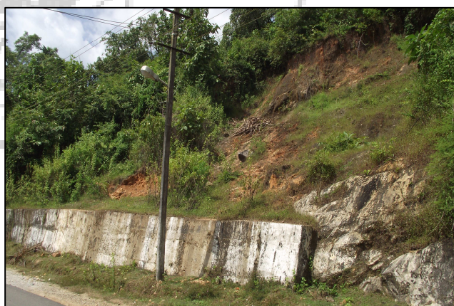
Photo 12: View of the landslide with toe wall constructed at facet 636 near Mundrali village
