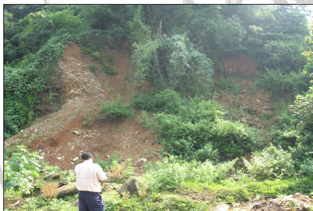
Photo 11: View of the landslide at facet 522 between Ankola - Karwar with gully erosion
