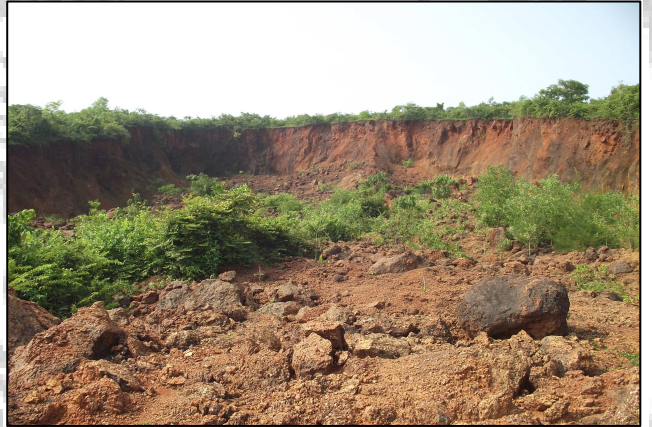
Photo 4: View of Kadwad landslide in which 19 people lost lives in facet no 606.
